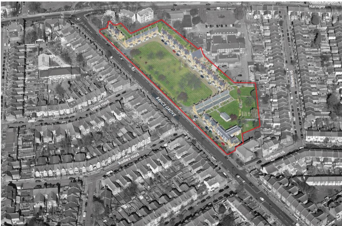
Fig 1. The site from above (looking north)
