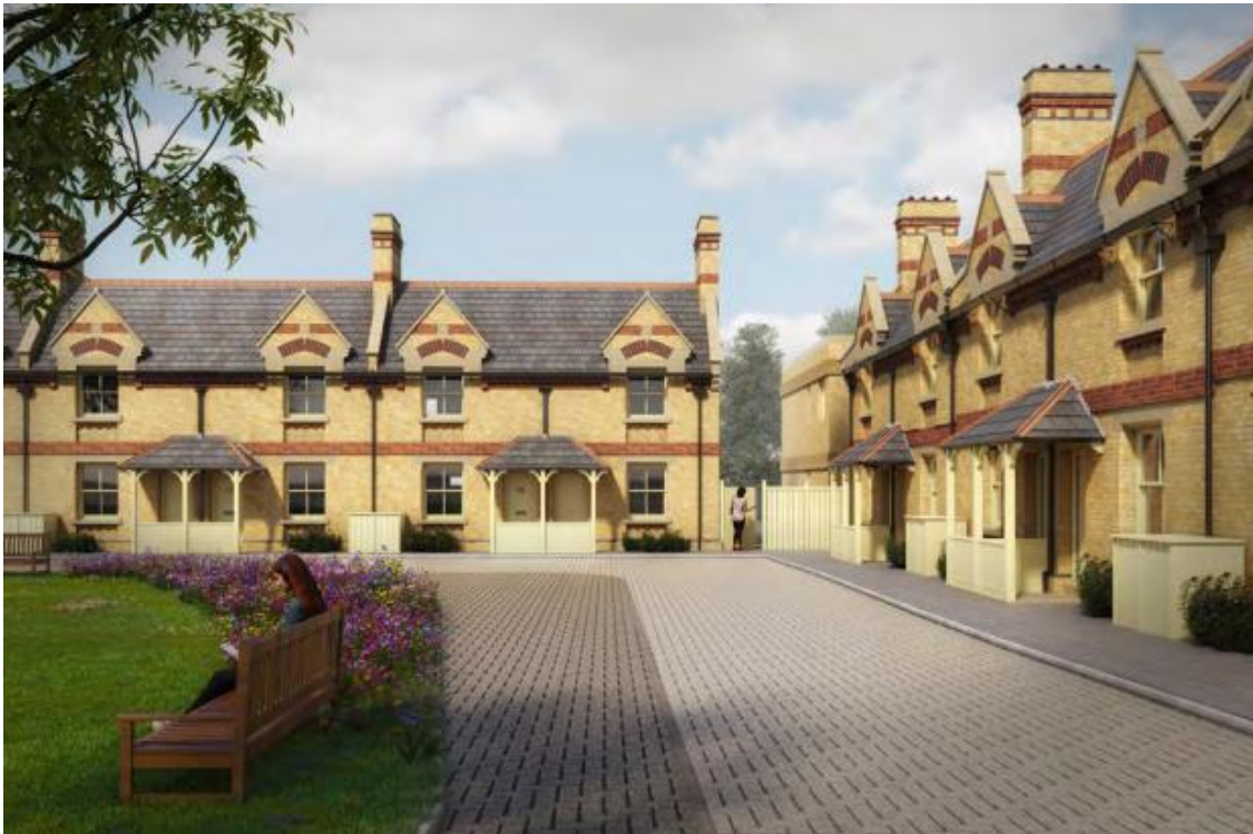
Figure 5 – 'Pavilion' extension when viewed from quadrangle.
